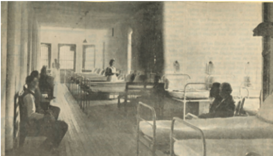
Figure 2 Hallway 7 of the Erie County Almshouse
